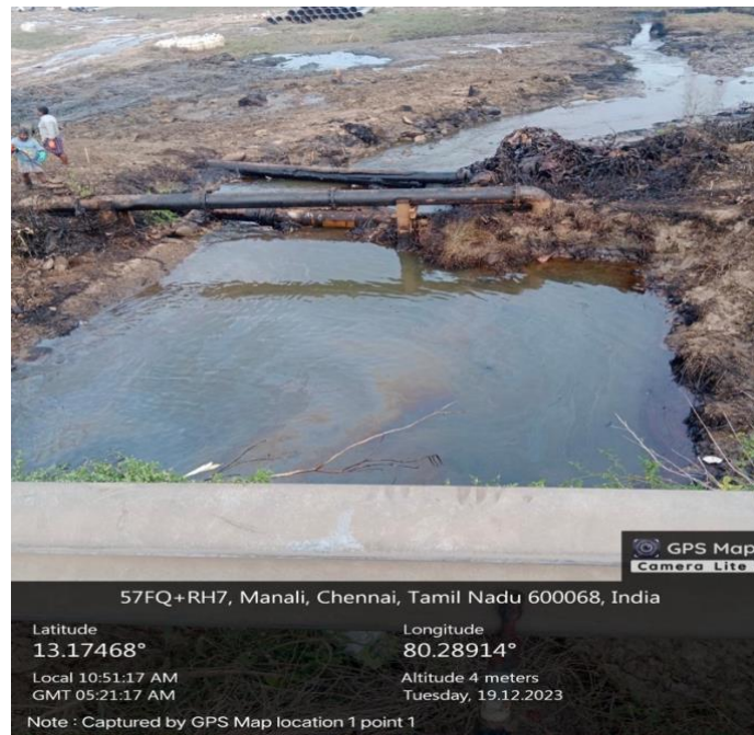
Figure 12: Close up view of Zone 1
