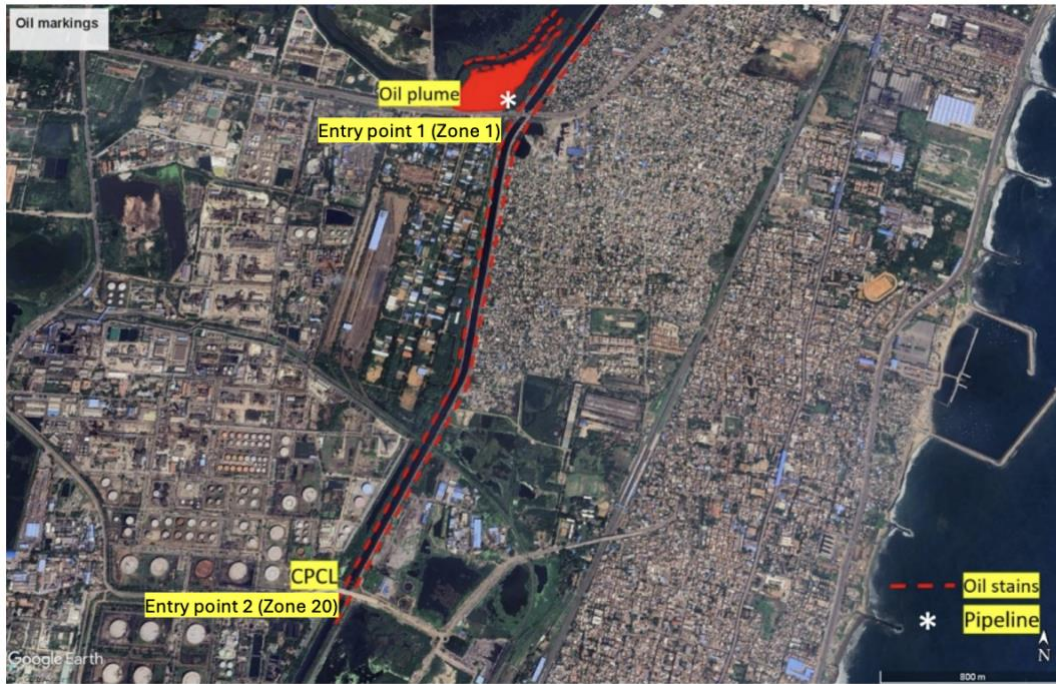
Figure 10: Assessment Region 3 - Upstream of B Canal from Manali High Road to Kodungaiyur showing the entry point of oil into the Buckingham Canal and Kosasthalaiyar River
