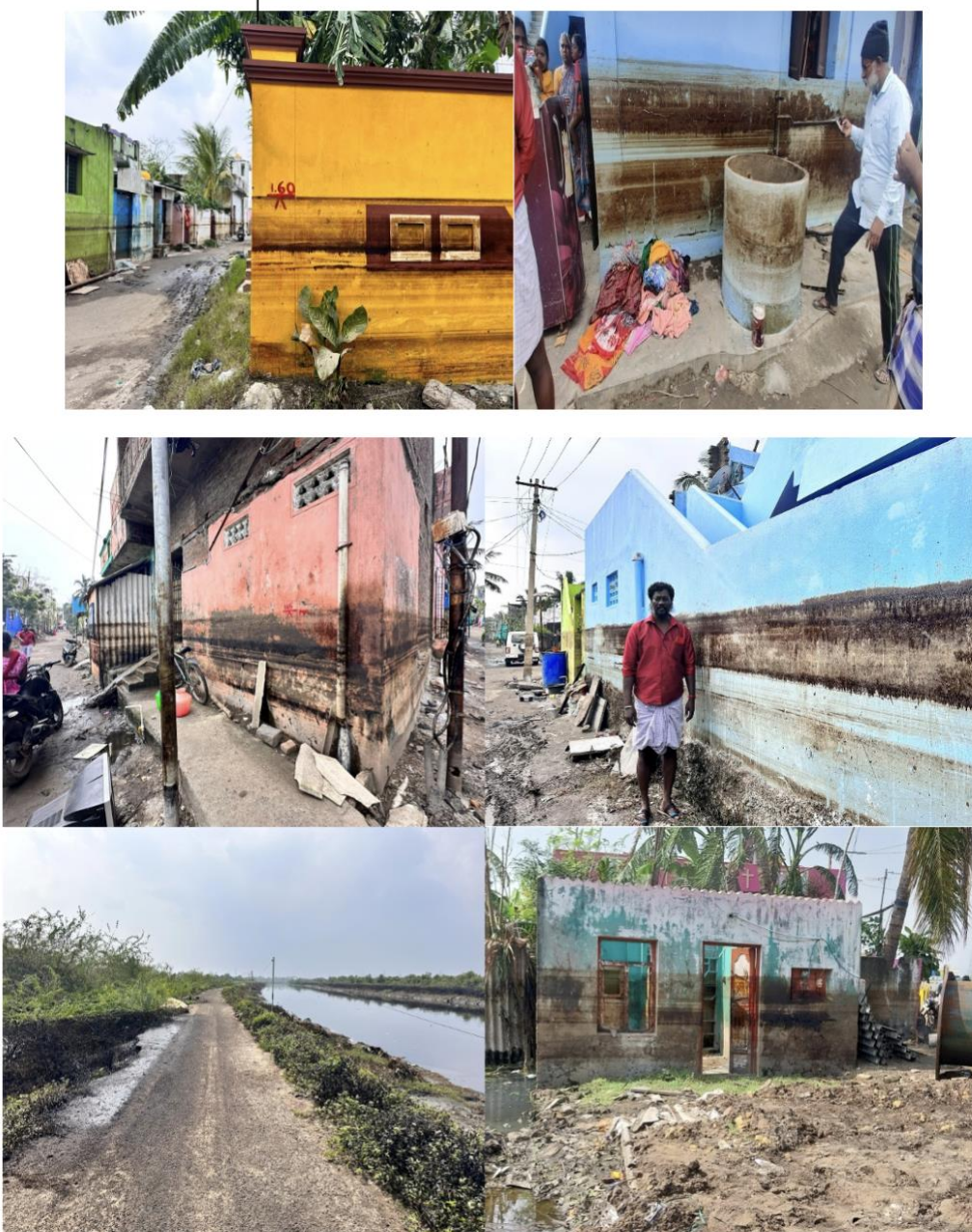
Figure 7: Oil marks observed in the residential localities of Ernavoor.
